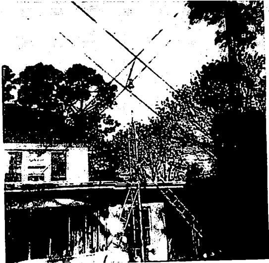
This new antenna, at the rear of the Greenwood home, will stand some 90 feet when completed. It is built to operate on a "directional pattern."
